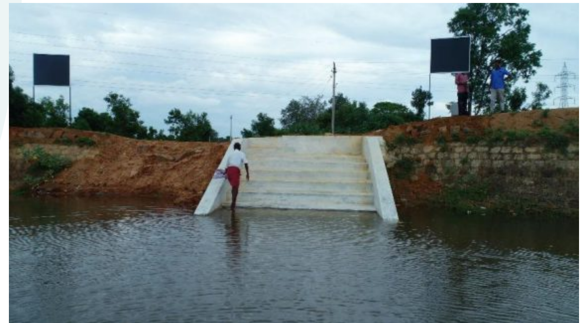
The steps were constructed to aid the communities
