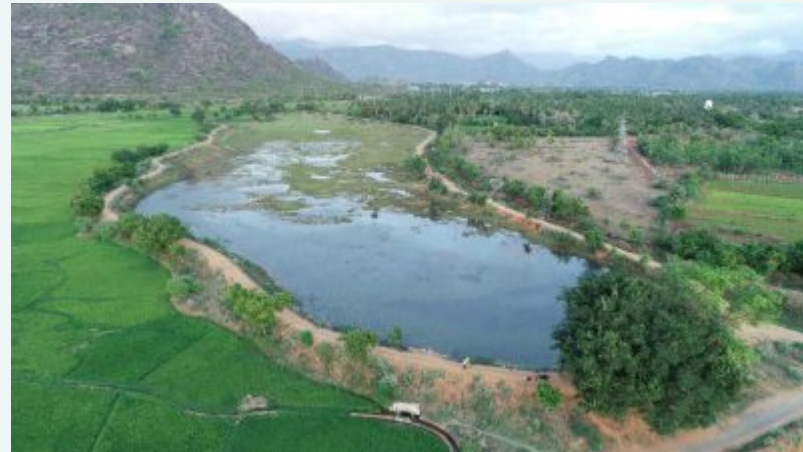
Aladikulam tank before restoration activities were undertaken
