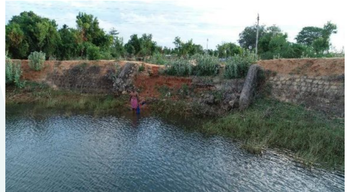
The steps before restoration
