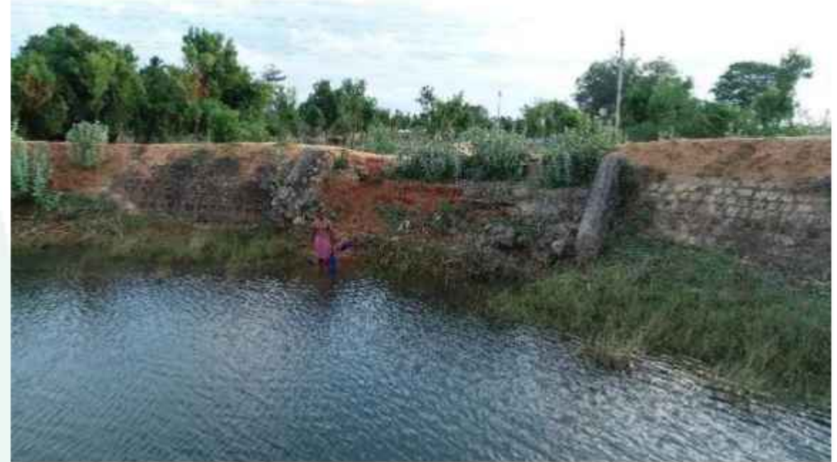
The steps before restoration
