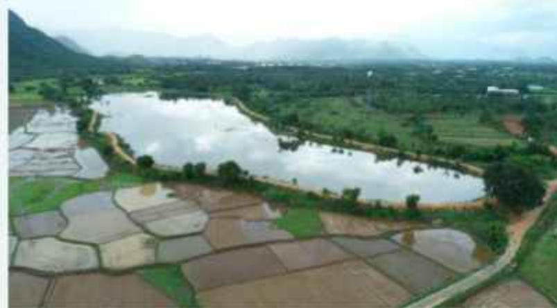
Aladikulam tank after restoration
