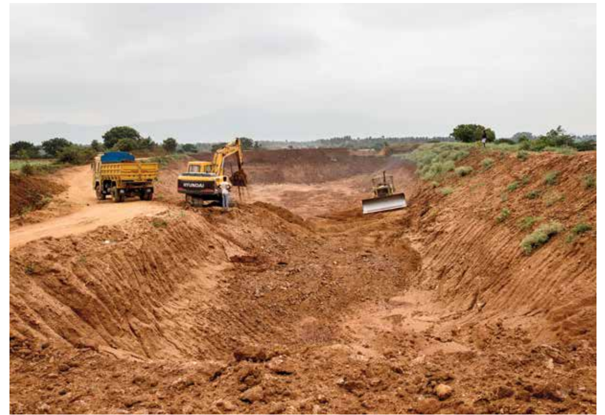
Clearing the river's path, bringing prosperity to the land
