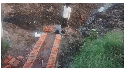
Construction of Inlet
