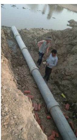
Installation of pipe
